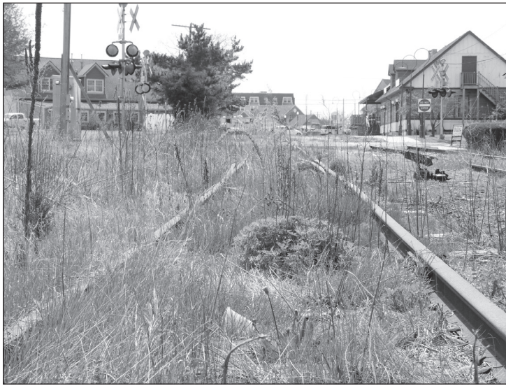
Jack Fichter/CAPE MAY STAR AND WAVE The city is considering expanding parking at the Welcome Center on long-unused train tracks adjacent to the building.
