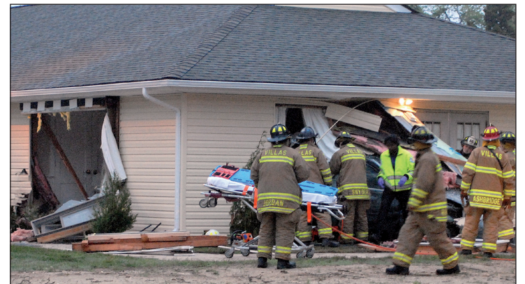
Robert Newkirk/Special to the CAPE MAY STAR AND WAVE Driver Kyle R. Crager-Hofferica, 31, of Villas, left the road and struck the building at about 5:45 a.m. May 14.
