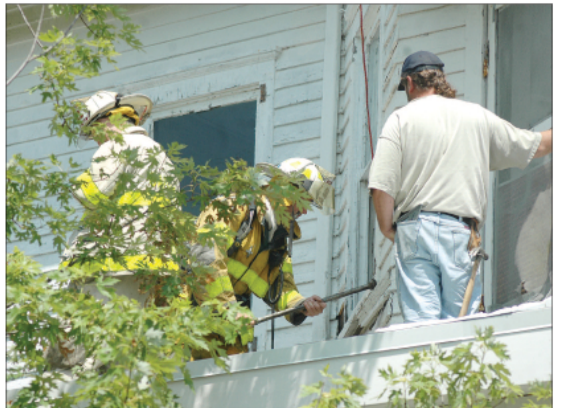
Cape May firefighters open a second floor wall at 201 Howard Street where workers accidentally ignited asphalt materials with a torch. Fire officials later discovered a number of fire code violations.
